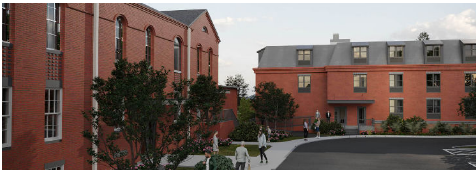
A new independent hotel with 95 rooms and suites is opening in the spring at the University of Maine. Hotel Ursa, inspired by the Ursa Major (the Great Bear) and Minor constellations and the North Star that connects them, was developed by renovating two of the oldest buildings on campus, Coburn and Holmes halls, and adding a new structure. Rendering of Hotel Ursa by Radnor Property Group.
